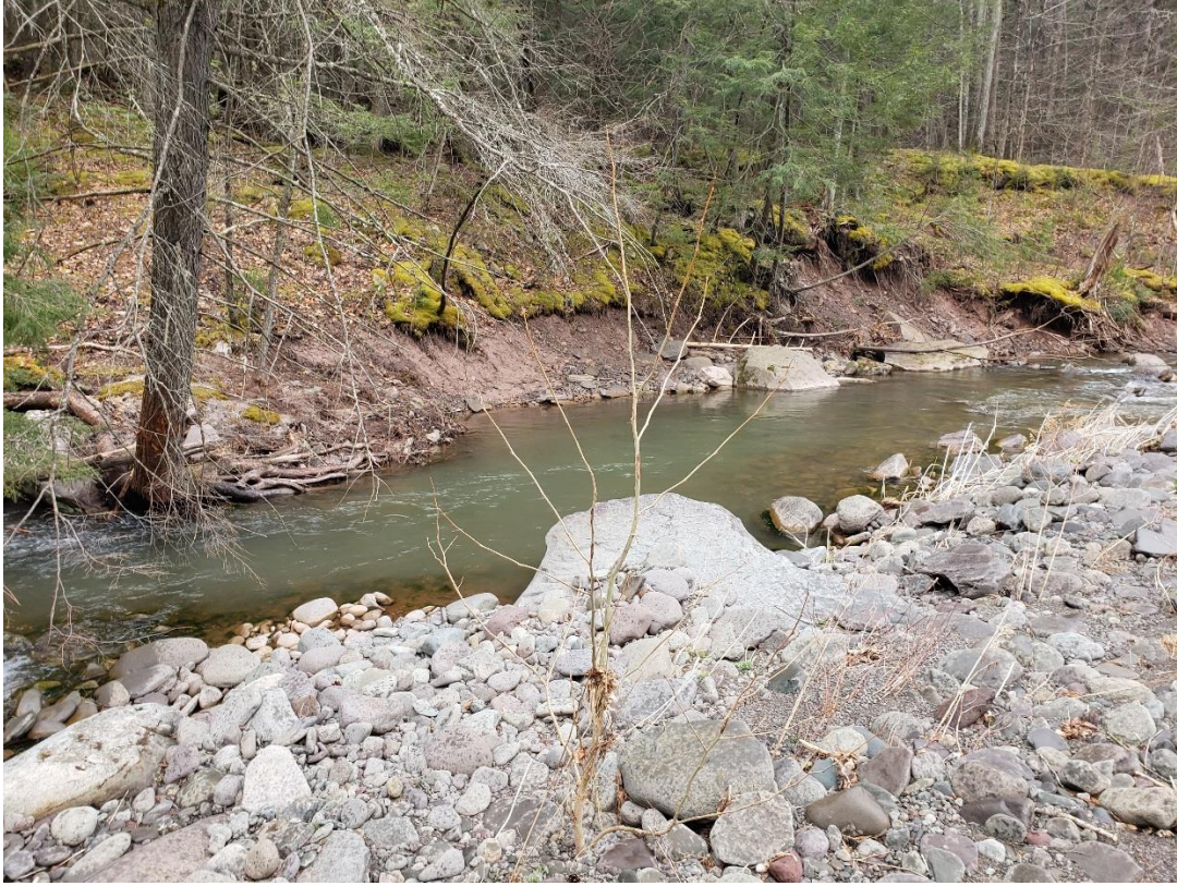
FIGURE 5. TOE EROSION, SLUMPING, AND ROTATIONAL FAILURE OF CLAY SLOPE.
